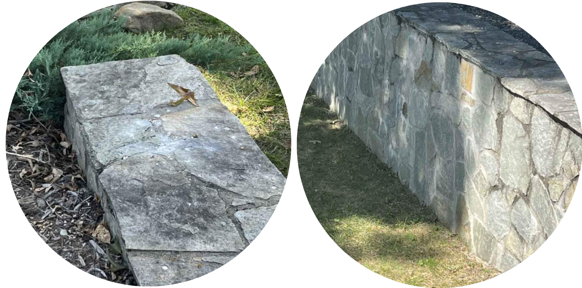
3 STONE VENEER RETAINING WALL MATCH EXISTING
