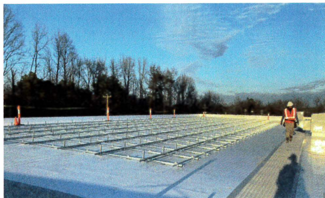
During Construction, February 2021
