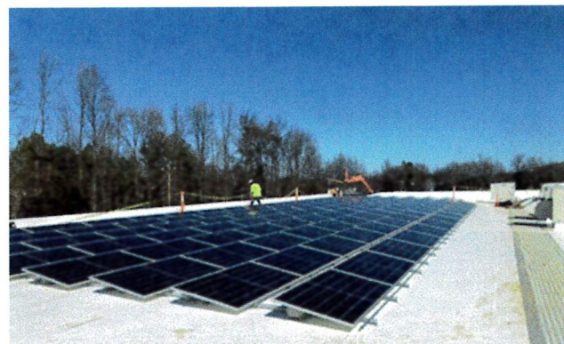
After Construction, February 2021
