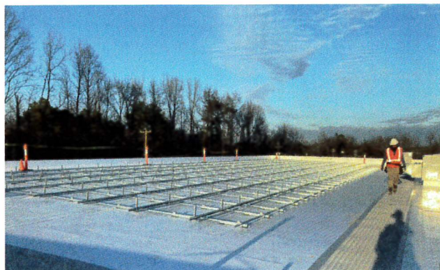
During Construction, February 2021
