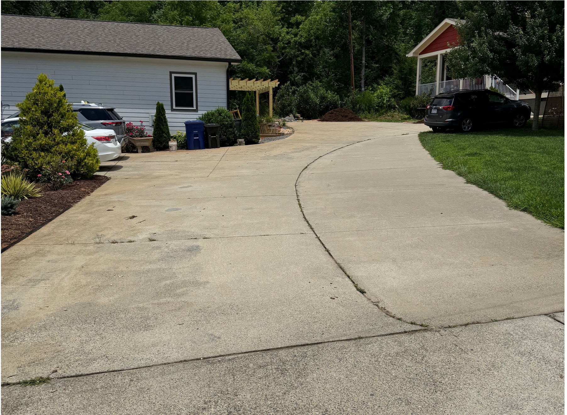
View from Shared Driveway Entrance to House
