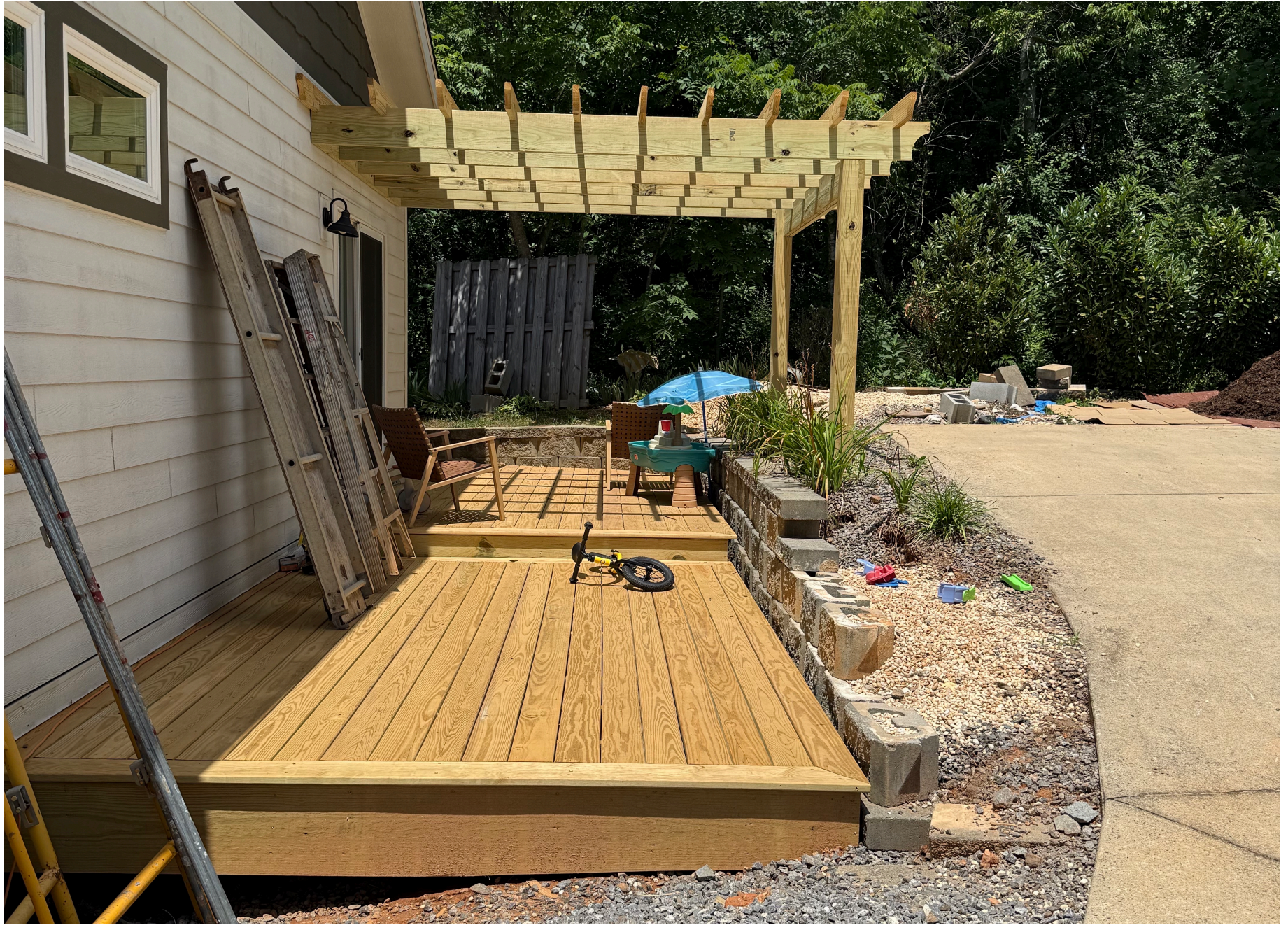
View of Rear Wall of House, Existing Deck, Retaining Wall, Pergola, & Neighbors Driveway
