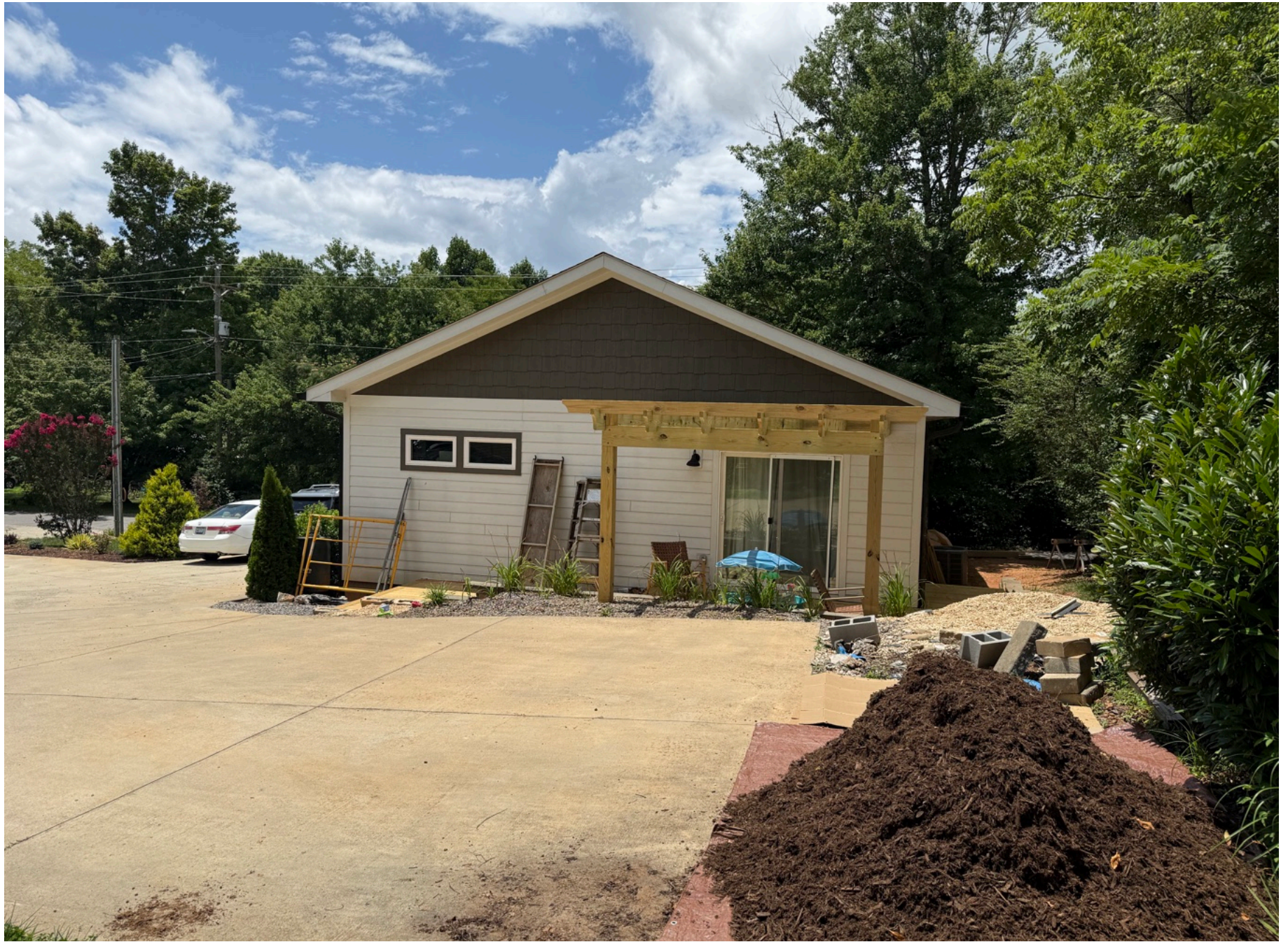
View facing the Rear Wall of House
