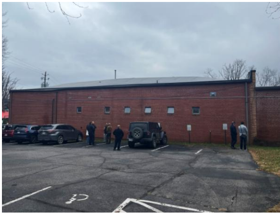
Photo 4: Police department roof.
