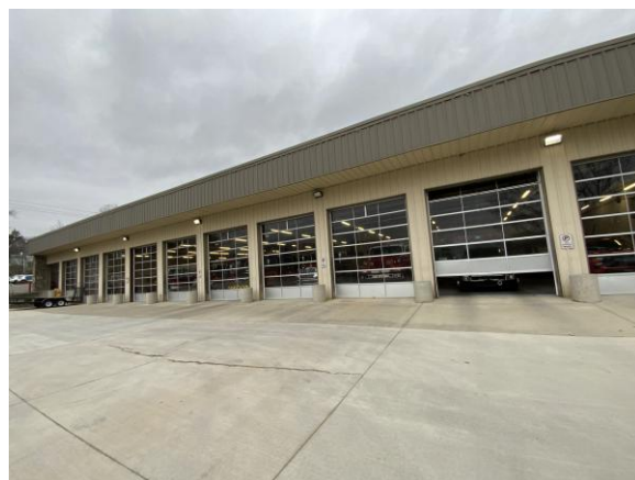
Photo 38: Apron in front of apparatus bay.
