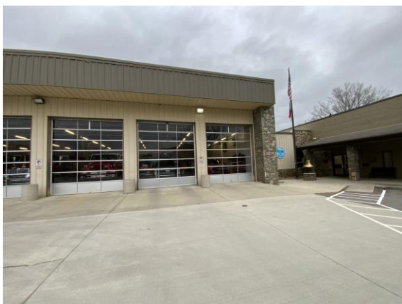
Photo 37: Apron in front of apparatus bay.
