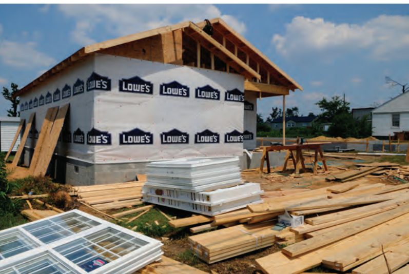
Rebuilding a residential home.
