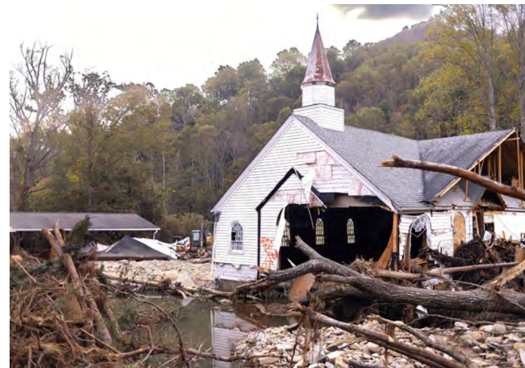
Damage to small church surrounded by vegetative debris.
