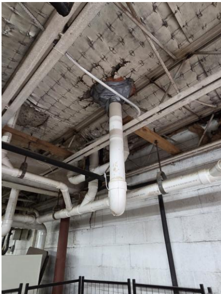
Photo 53: Patched sanitary waste piping.
