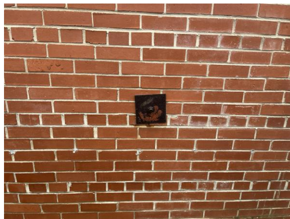
Photo 4: North wall tie.
