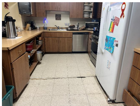
Photo 11: Fire station kitchen VCT floor.
