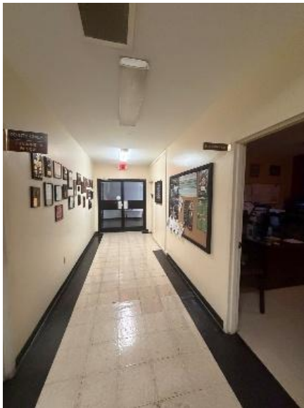
Photo 49: Typical light fixture.
