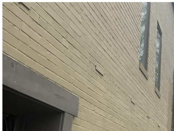
Photo 2: Closeup of east wall.
