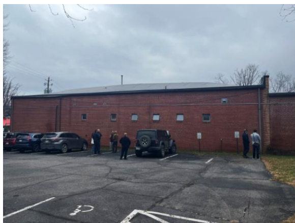
Photo 5: Police department roof.
