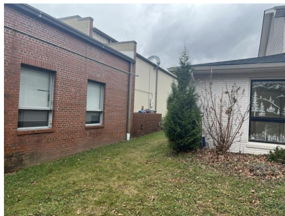
Photo 8: Windows on north side of building.
