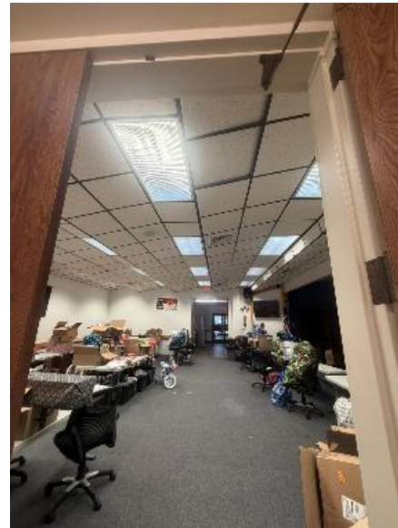
Photo 48: Typical light fixture.
