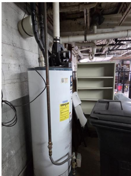
Photo 56: Basement water heater.
