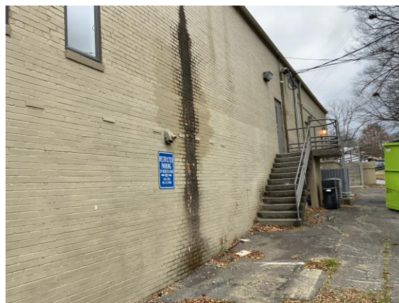
Photo 6: Missing downspout.
