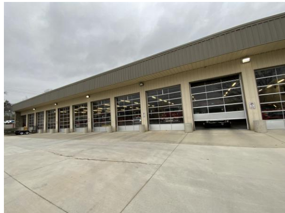
Photo 105: Apron in front of apparatus bay.
