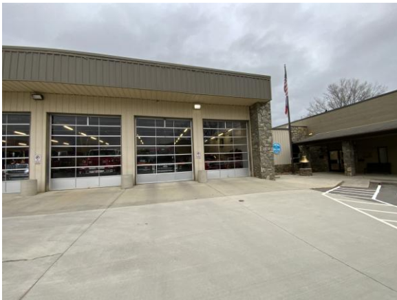
Photo 104: Apron in front of apparatus bay.
