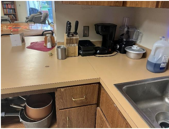
Photo 12: Fire station kitchen casework.
