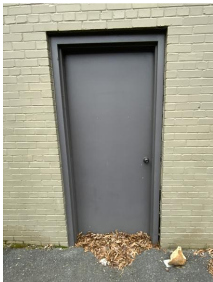
Photo 9: Exterior door on east side of building.
