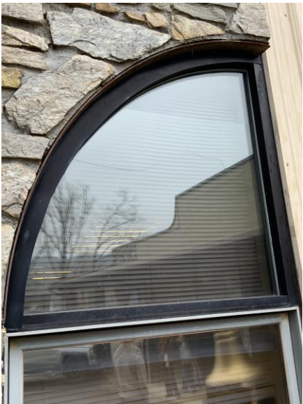
Photo 98: Cracked window.
