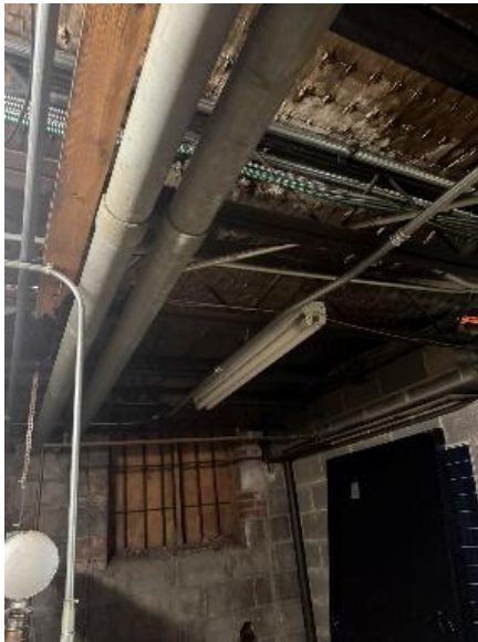
Photo 47: Typical light fixture.
