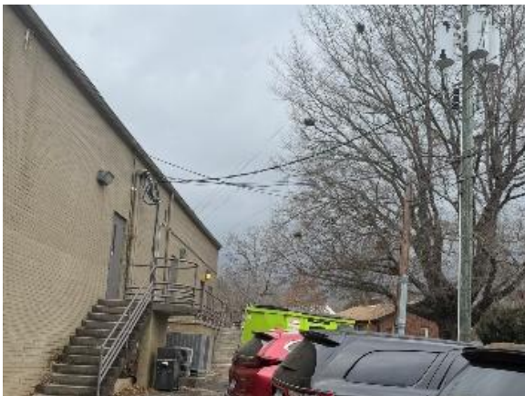
Photo 39: Utility power pole.
