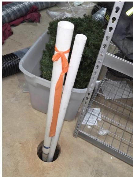
Photo 58: PVC drain pipes.
