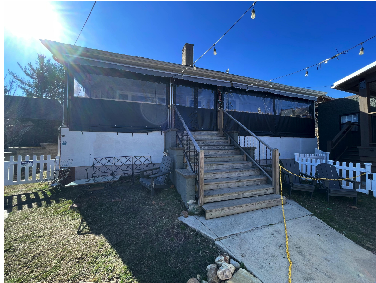
EXISTING STREET FACADE
